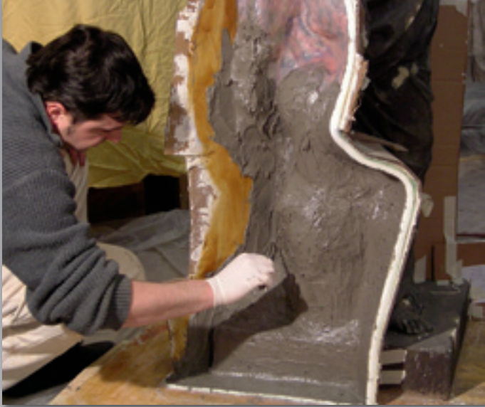
12 | Application du mastic Epoxi GF
