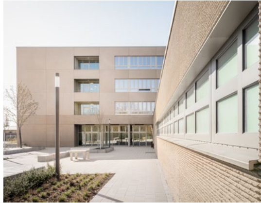
▲ The integrated secondary school for up to 725 pupils was built in the growing Berlin district of Lichtenberg.
