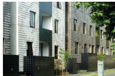
Residential building façade
